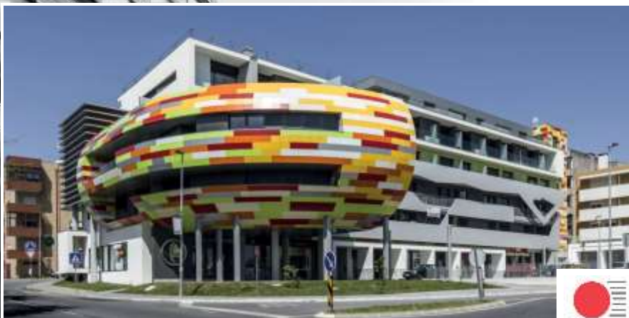
STAC BOND - Composite Panel - Hospital de Lourenço - LISBOA
