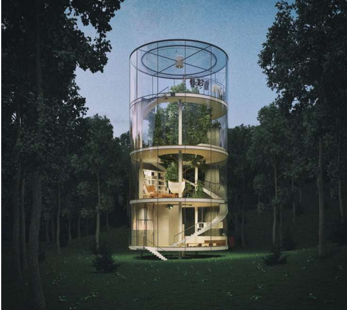
A. Masow Architects, Tree in the House , Kazakhstan, 2013.
