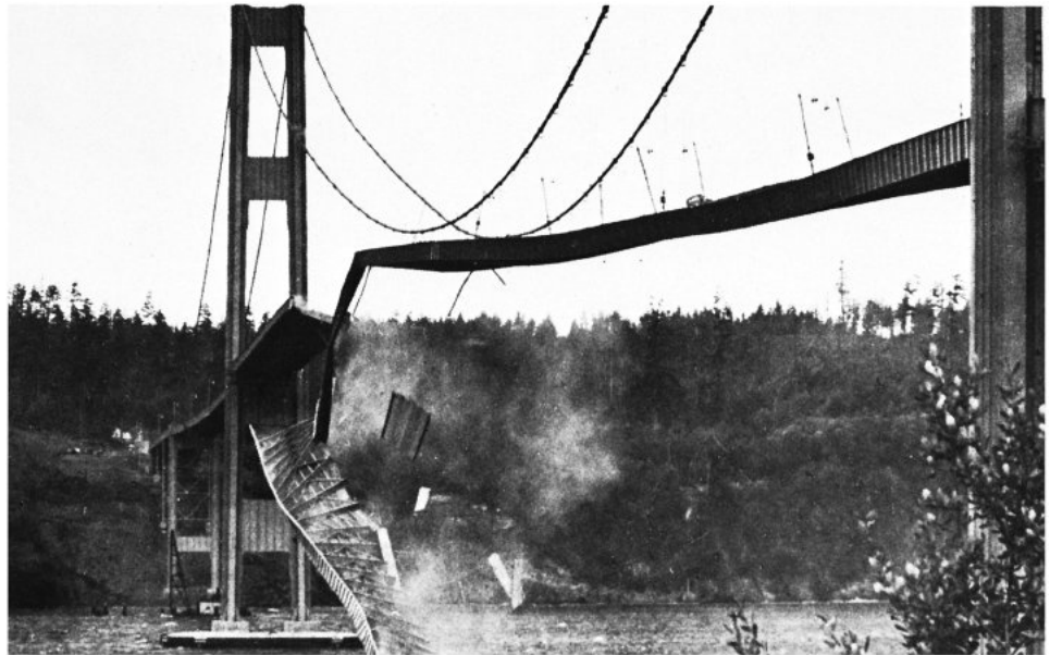
FIGURE 1.7 Tacoma Narrows bridge during wind-induced vibration. The bridge opened on July 1, 1940, and collapsed on November 7, 1940. (Farquharson photo, Historical Photography Collection, University of Washington Libraries.)
