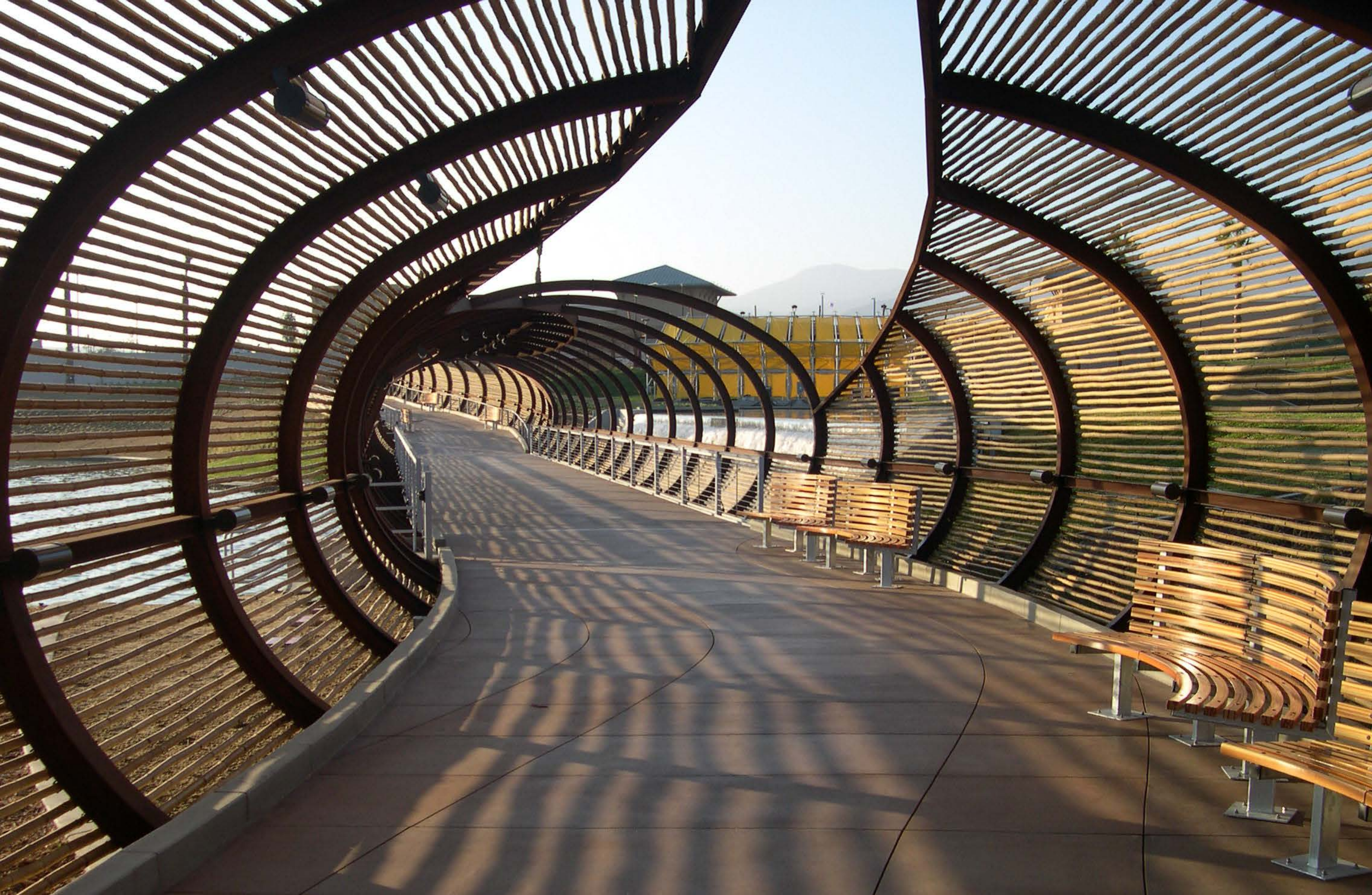
Walkway in Corona, CA. made of 93% Recycled steel and bamboo
