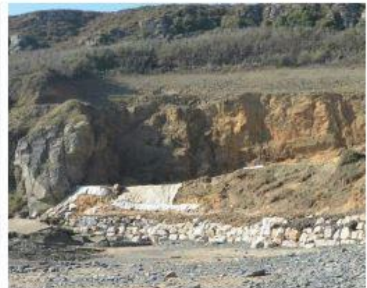
Fig. S4. View of Le Rozel site: during the first excavations in 1969 (left) and in 2014 (right). The riprap at the base of the dune was built in order to limit the tidal sapping action
